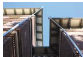
Seminaarinmäki campus is a valuable entity due to its architectural, cultural and horticultural history. The oldest buildings date back to the 1880's.
